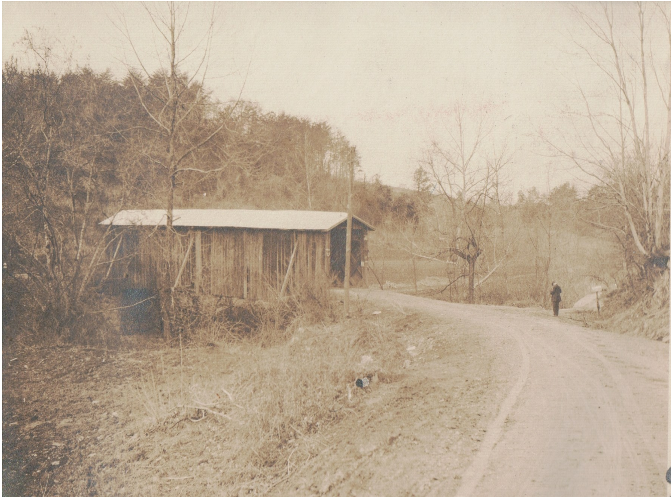
Old Covered Wooden Bridge over Buffalo River on the road to New Glasgow (P.O. Clifford)
