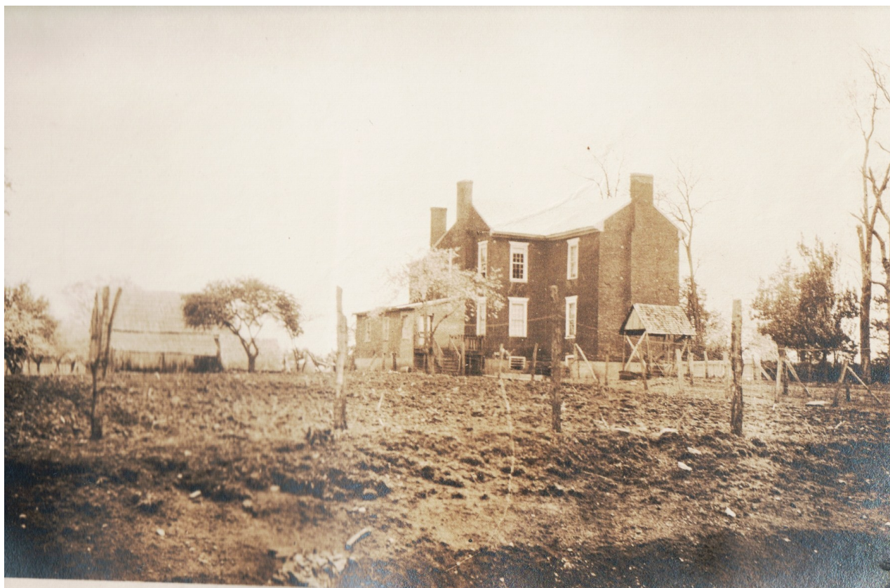
Rear view of Pendleton house.
