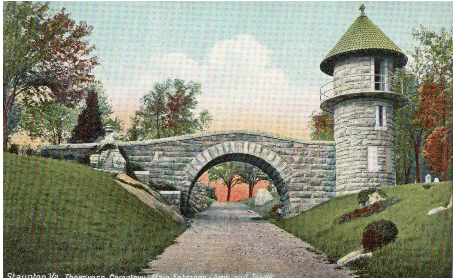
Staunton, Va., Thornrose Cemetery-main Entrance-Arch and Tower
